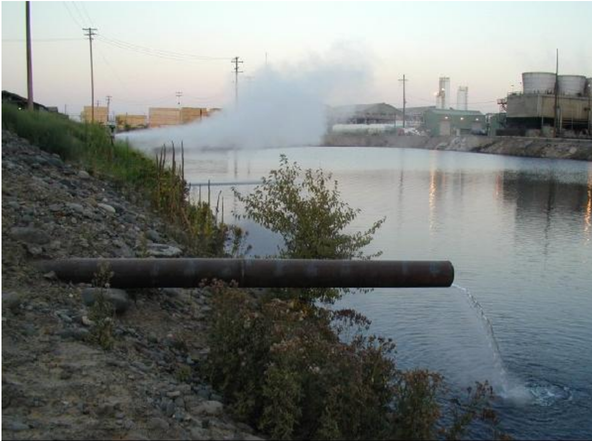
Discharge from kilns with Enercon Systems units (foreground). Discharge from bucket traps (background)
